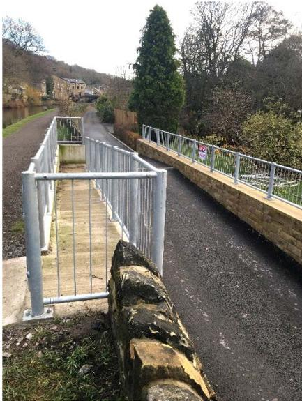
The canal access ramp is now complete with hand railing installed (image left). This provides an escape route to the canal towpath for residents of Tillotson Holme and the bowling club during flood conditions. The escape route is a private access and not open for public use.
