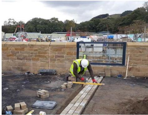
Reinstatement of the area next to Barbary's is underway (image left). Glass panels have now been installed in the flood wall and a raised planter has been constructed. Stone paving and a resin bound finish will be laid next, and a bench installed.
