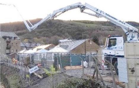
The concrete pour for the foundations of the new flood defence walls was completed last week using a 45 metre concrete pump.
