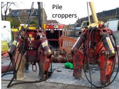
The piles were temporarily cast to ground level to protect the bars from damage by the heavy plant during the earlier piling works and also to maintain the integrity of the piles below final cut off level.
