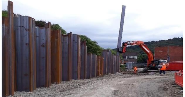
Piling works continue with 102 out of 132 piles now in place. These piles will facilitate the widening of the channel and will be back-driven to the correct height. We will continue to monitor noise and vibration levels throughout the work. On completion of piling these will be clad with natural stone.
