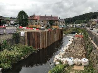
Piling work will shortly commence on the right bank to enable construction of the northern pier for the new bridge.
